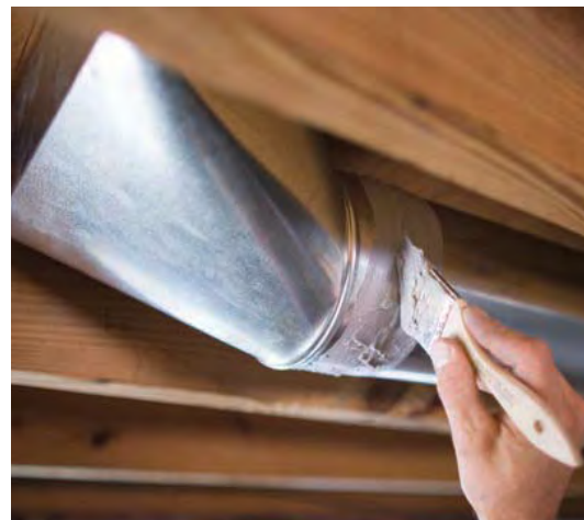
Sealing ducts in your home can help improve the overall efficiency of the air conditioner.
