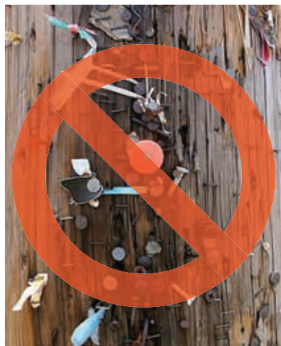
Attaching signs to power poles creates serious safety hazards.
