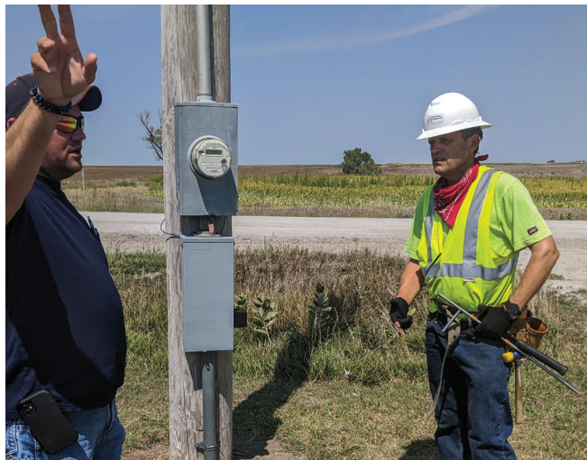
Western Line Superintendent Ron Aschenbrenner (left) discusses pole testing procedures with Utility Asset Management President Wayne Hall.
