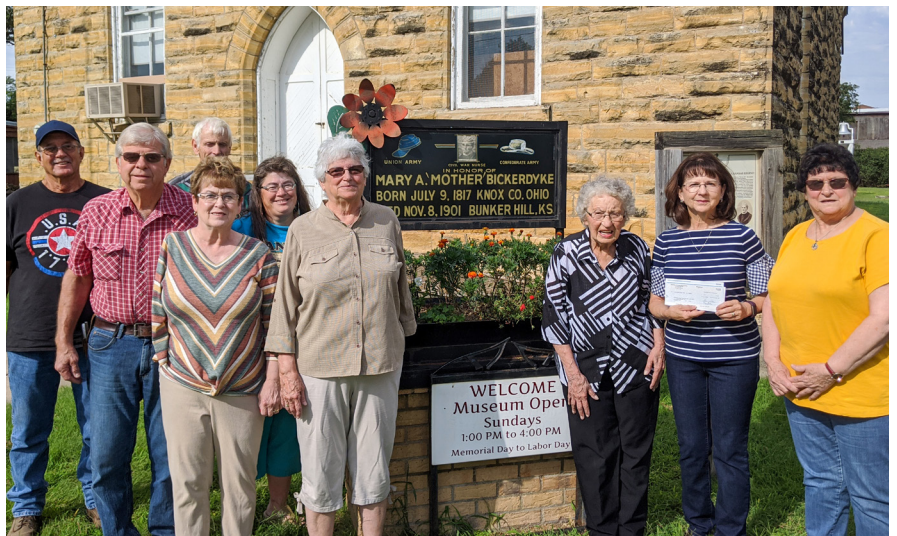
The Bunker Hill Historical society replaced a non-functioning bathroom with an ADA-compliant bathroom facility for their museum.
